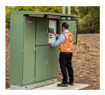
The Global Water range of Kwikstart™ alarm panels have been developed to provide a level alarm warning in septic tanks, water storage tanks, pump sumps and dump pits.
