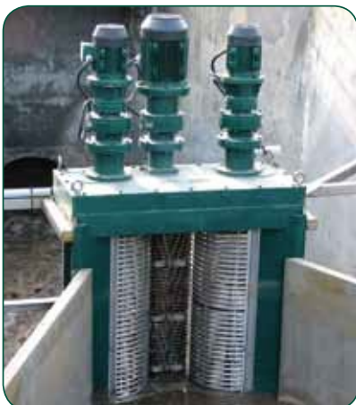
Wastewater entering a Channel Monster grinder.
