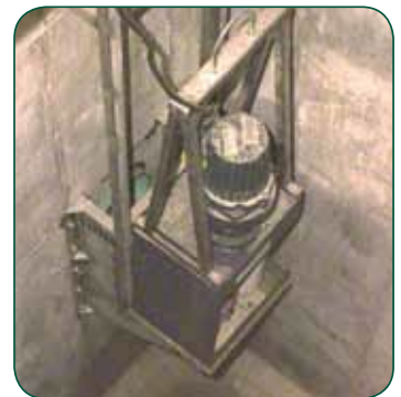
Channel Monster in a pump station with custom guide frames.
